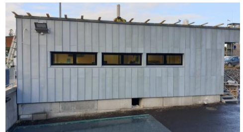
New zinc facade made of reused RHEINZINK from Kiasma.
