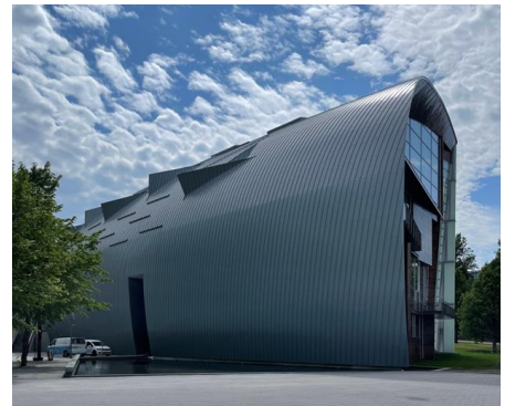
The same expression with the new RHEINZINK façade – but now with an internal renovation for more energy efficiency.
