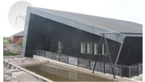
The new visitors building with details in RHEINZINK reused from the Kiasma Museum façade cladding.
