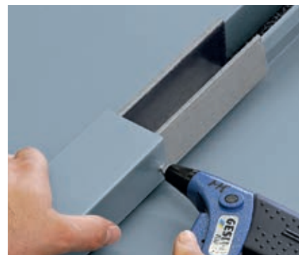
Fig. 18: Installation of rivet
