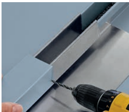
Fig. 17: Drilling a hole for the rivet
