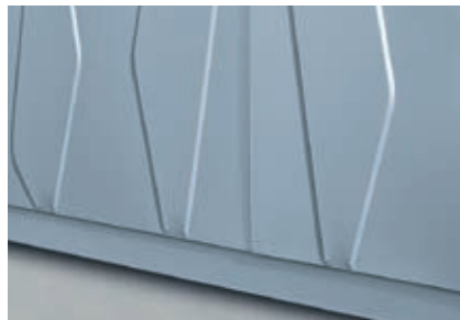
Base connection The crystal tiles are suspended in the prefabricated base profile.
