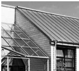
Fig. 13: Pent roof ridge with timber batten
