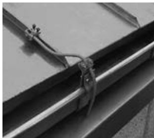
Fig. 9: Proper installation allows for thermal expansion of panel
