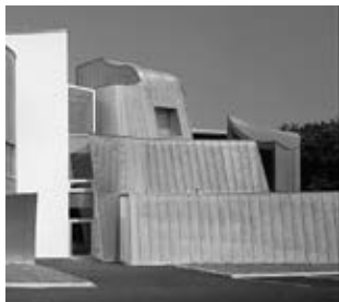
Fig. 1: RHEINZINK-prePATINA bright rolled surface, VITRA Administrative Building in CH-Birsfelden
