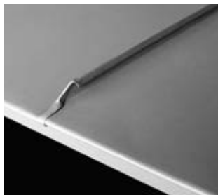
Fig. 14: Ridge as eave termination
