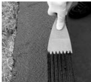
Fig. 4: Apply Enkolit® with notched trowel
