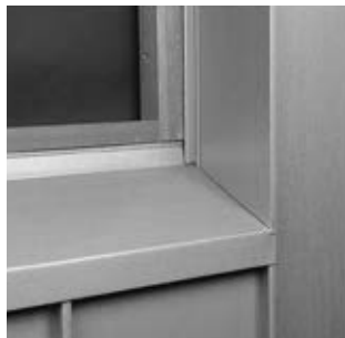
Fig. 21: Jamb on lateral connection windowsill coping
