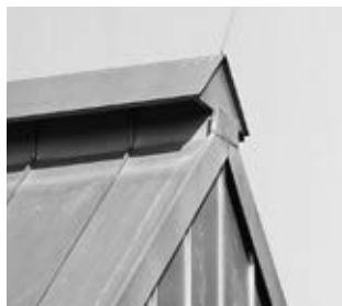
Fig. 11: Flush ridge termination on verge, high design
