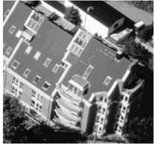
Fig. 27: Attic – cornice copings
