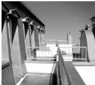
Fig. 26: RHEINZINK flashing as a wall coping
