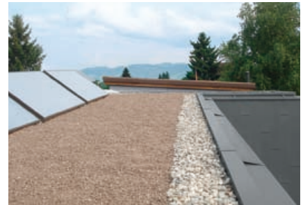
Flat roof with solar collectors, edge termination and tile facade
