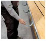
Locate the gutter brackets at a maximum spacing of 90 cm.
