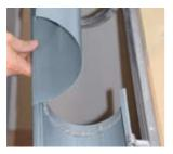
Twist gutters inside each other. Ensure a gutter overlap of 50 mm.
