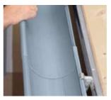
Wipe off any adhesive emerging with a cloth. Gutter corners are bonded in the same way.
