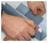
Stick 2 strips of adhesive tape approx. 20 mm long (e.g. 3M<sup>®</sup> type 4950F) on the outside corners of the expansion element, remove backing film.
