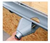
Hook the plug-in outlet into the gutter bead.
