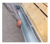
Fasten the gutter by snapping the gutter bead onto the snap-lock bracket.
