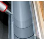
Apply adhesive onto the gutter bead, on one gutter section only!
