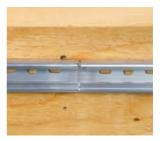
Mount adjacent rails with a gap of 3-5 mm to accommodate linear thermal expansion.
