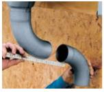
Determine the length of the piece of straight pipe so that the vertical section of downpipe is a minimum of 20 mm from the wall.
