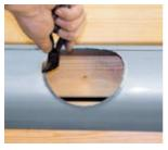
Create a drip edge by bending a 5 mm edge toward the outside of the gutter.
