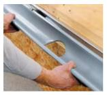
Snap the gutter bead onto the nose of the snap-lock bracket at the front.
