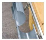
Join the gutter pieces with an overlap of 50mm, without using adhesive! twist in the gutter bead...
