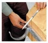
Start the installation by locating the highest point of the gutter. The extension of the roof surface (see pencil in illustration) should extend into the gutter.
