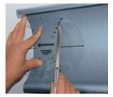
Mark the second half of the opening for the gutter outlet, offset 50mm to the inside.
