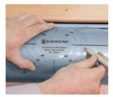
Mark the exact location of the cut out using the RHEINZINK Gutter Outlet Template. Align the centerline of the template at the lowest point of the gutter.
