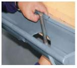
Bend strips downwards and create a 10 mm water check along the opening.
