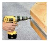
Fasten the snap-lock fixing rail with a slope of 1-3 mm/m. Mount the rail with the longer leg at the bottom.
