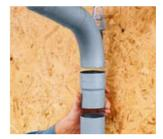
Insert the downpipe adaptor with the expanded end toward the top.
