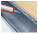
Apply 2 beads of adhesive – min. diameter 8 mm – each approx. 25 mm away from the edge of the expansion element on the inside.
