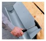
Drive-in the roofing nails at staggered locations at horizontal intervals of 100 mm.
