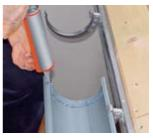
Remove dust and grease from gutter parts to be attached. Apply bead of adhesive – min. diam. 8 mm – approx. 25 mm from the end of the gutter.
