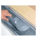
Stick in expansion element so that it is rigid, press corners firmly to the adhesive tape.
