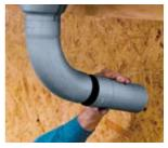
Insert expanded end of the downpipe over the pipe bend...
