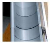
Roll the gutter bead cap over the edge of the expansion element. The cap prevents rainwater from getting in between the expansion element and the gutter.
