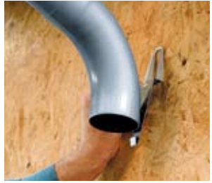
Hook in the Universal Downpipe Bracket.
