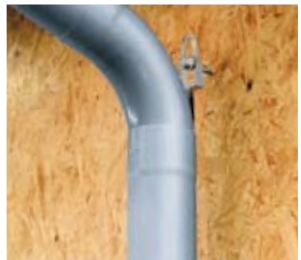
Connect the next downpipe component by sliding on the expanded pipe end.
