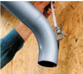
Fasten the Universal Downpipe Bracket onto the screw.
