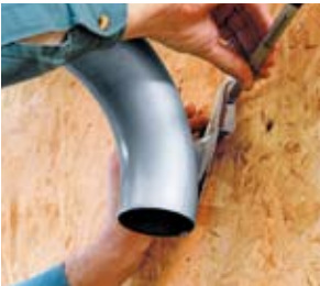
Mark the position of the screw.
